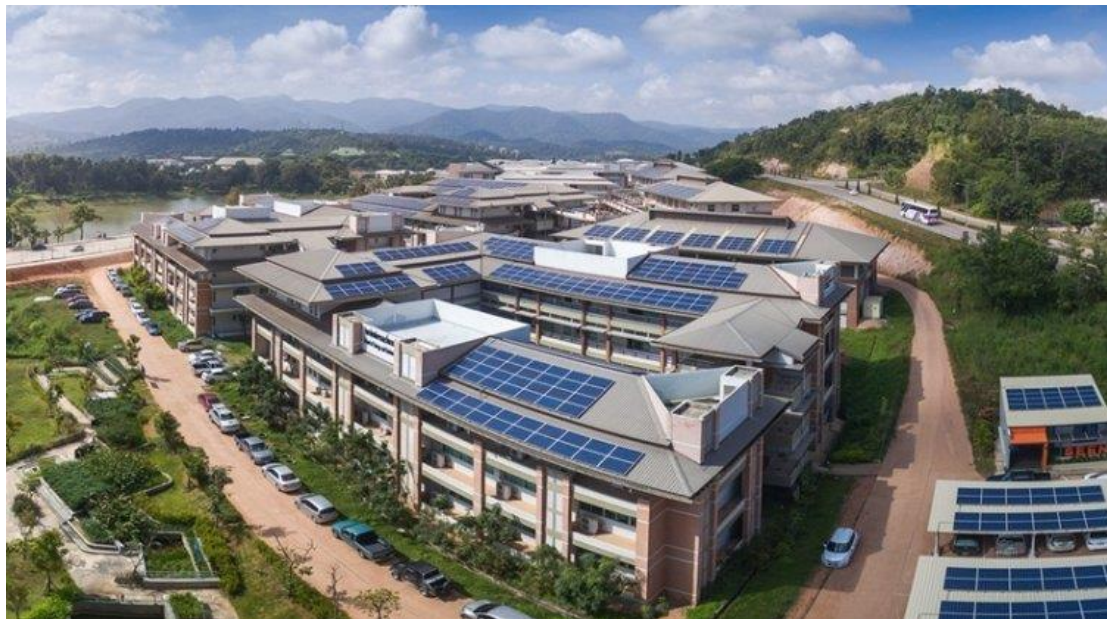
Roof Solar Panels (University of Phayao, Thailand)
